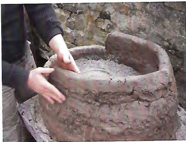
Building the sand-filled oven
